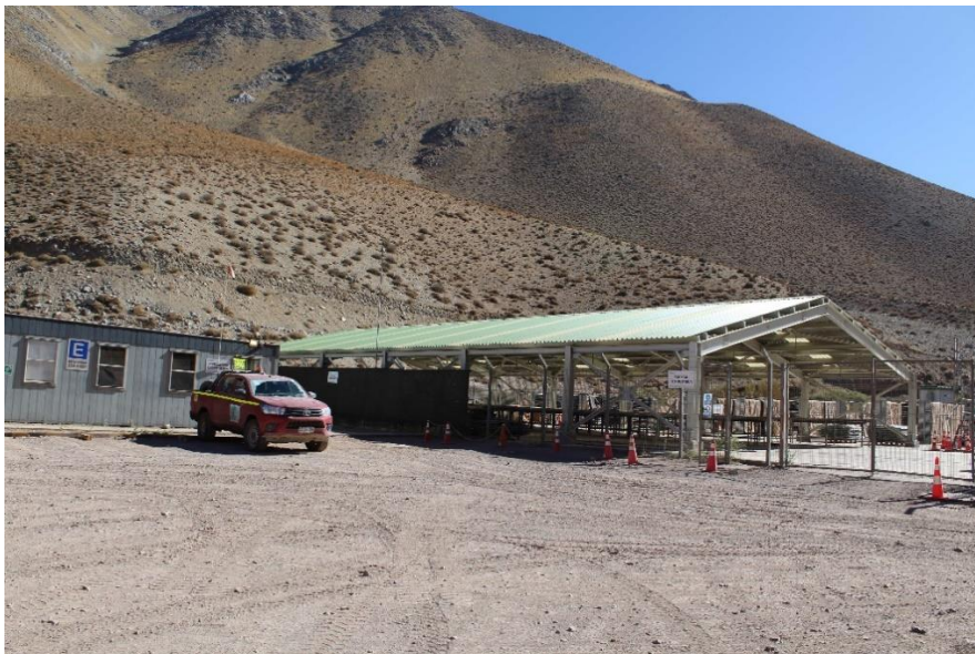
Figure 12-3: Centre Administrative (left) and Core Shack (right)
