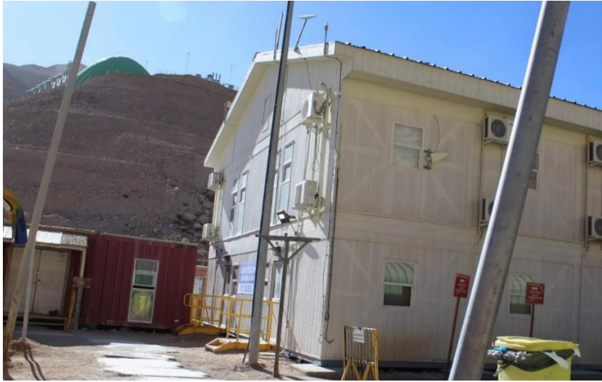
Figure 12-5: Mine Office Facility
