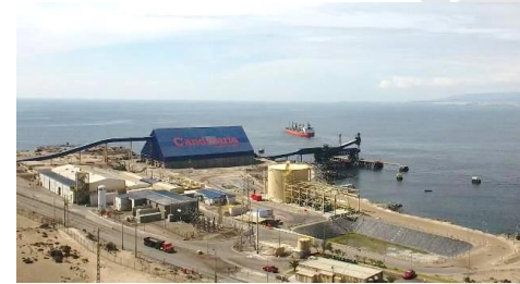
Punta Padrones Port and Desalination Plant, Caldera
