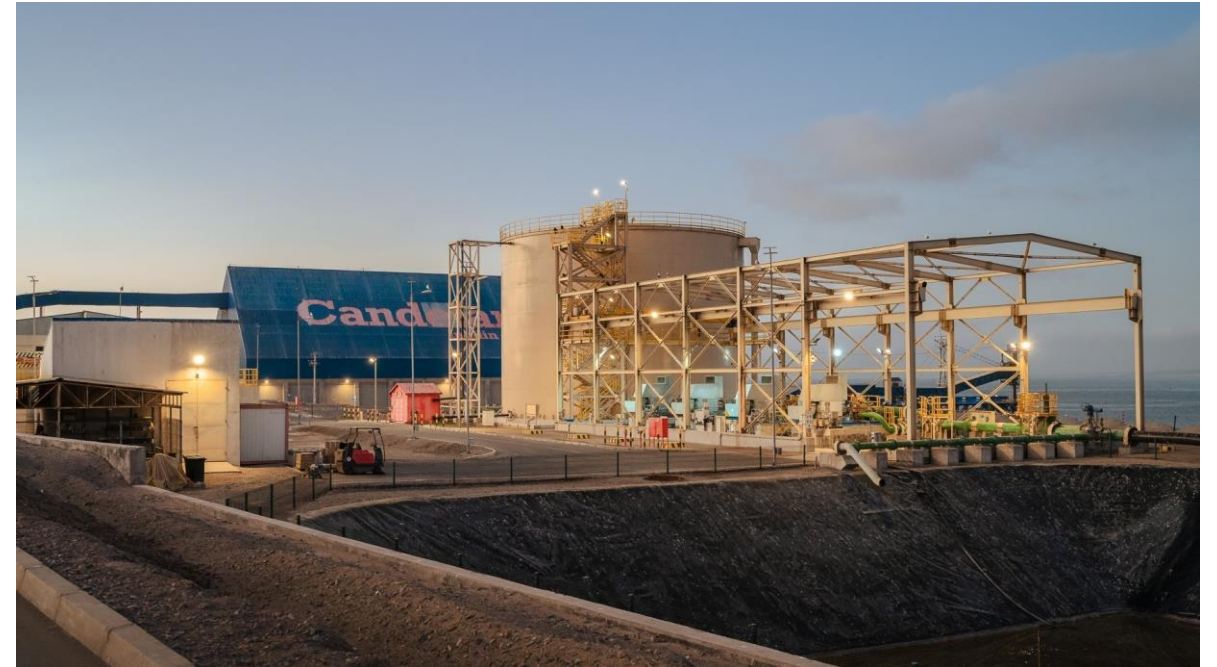
Candelaria, Punta Padrones Port & Desalination Plant, Chile
