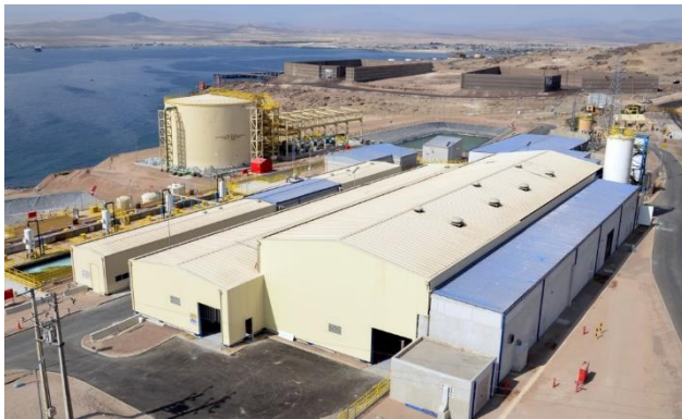
Candelaria desalination facility
