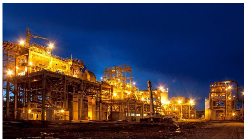
Chapada processing plant
