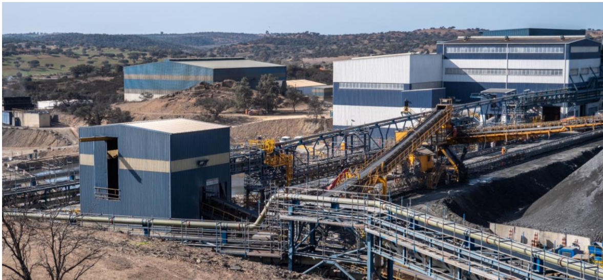
ZEP surface facilities – February 2022
