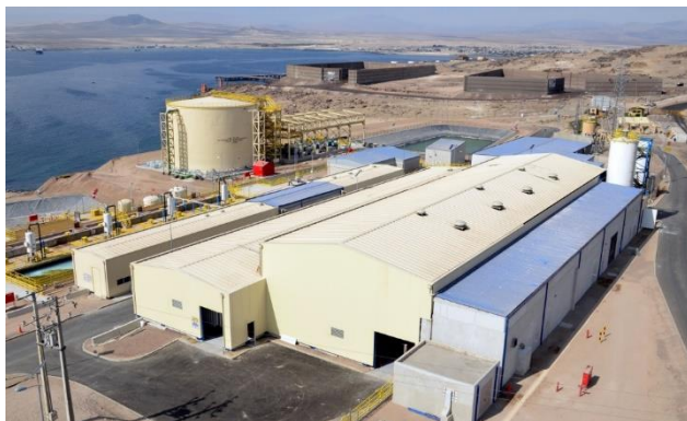
Candelaria desalination facility
