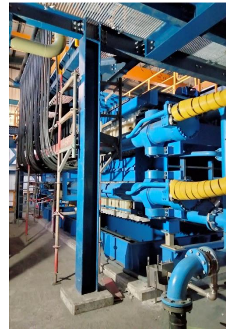
Zinc filtration works complete
