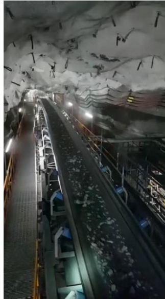
Material handling system commissioning
