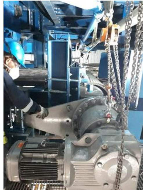
Zinc filtration drive system and filter press works
