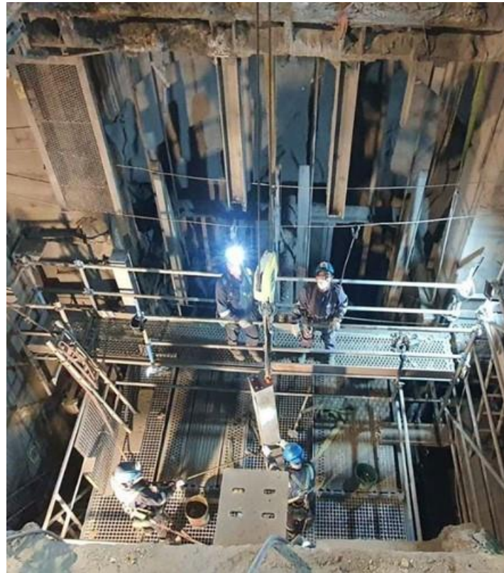
ZEP shaft upgrade mechanical works – August 2021
