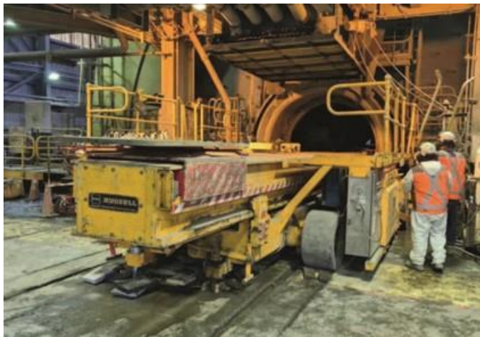
Maintenance on Line 2 of Concentrator – September 2021
