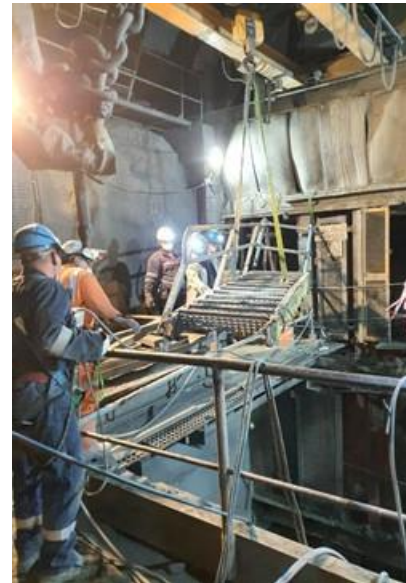
Shaft upgrade mechanical works
