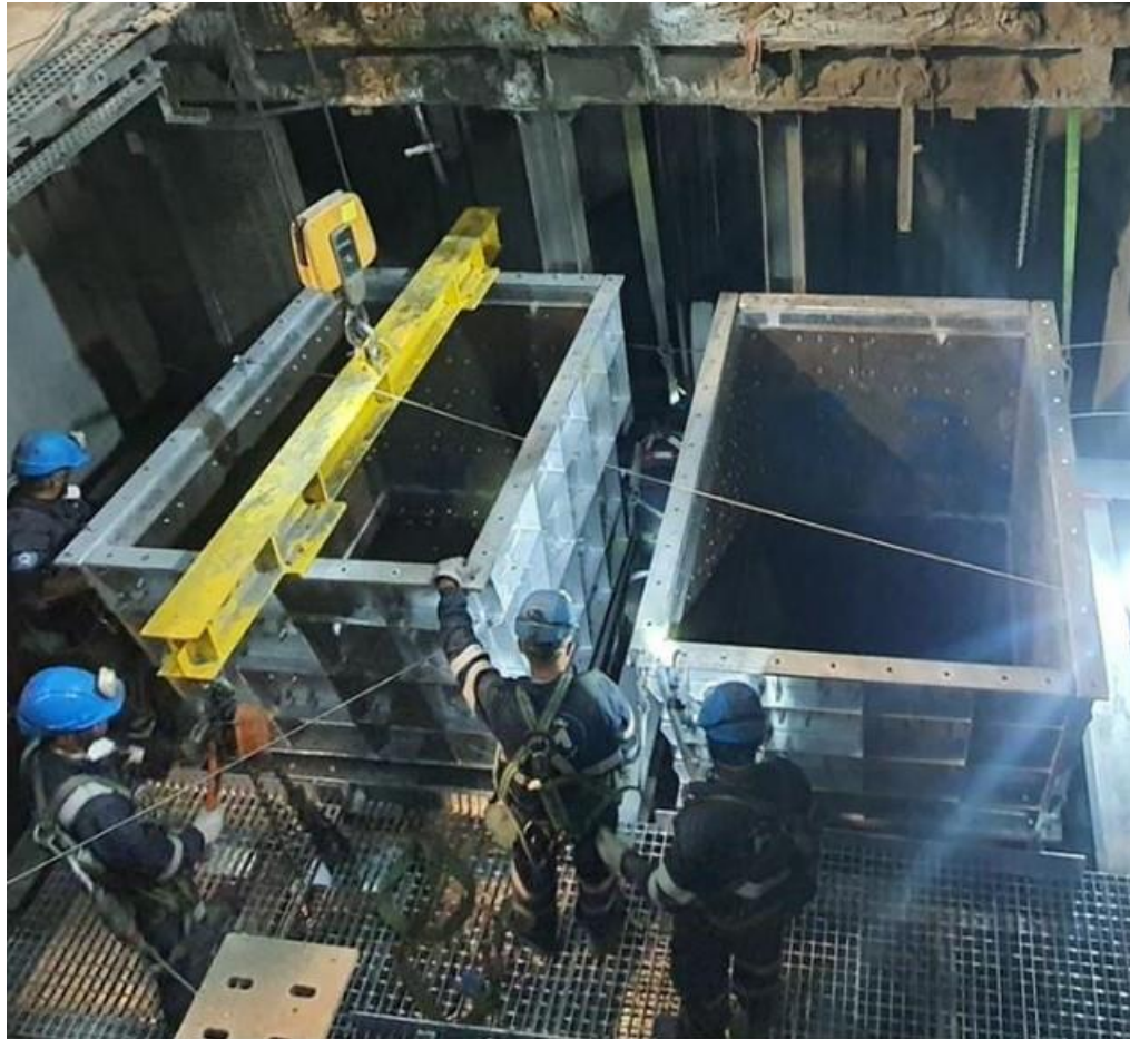
Neves-Corvo ZEP shaft upgrade work – August 2021
