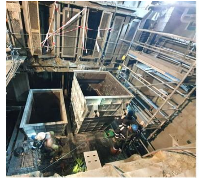
Shaft upgrade construction
