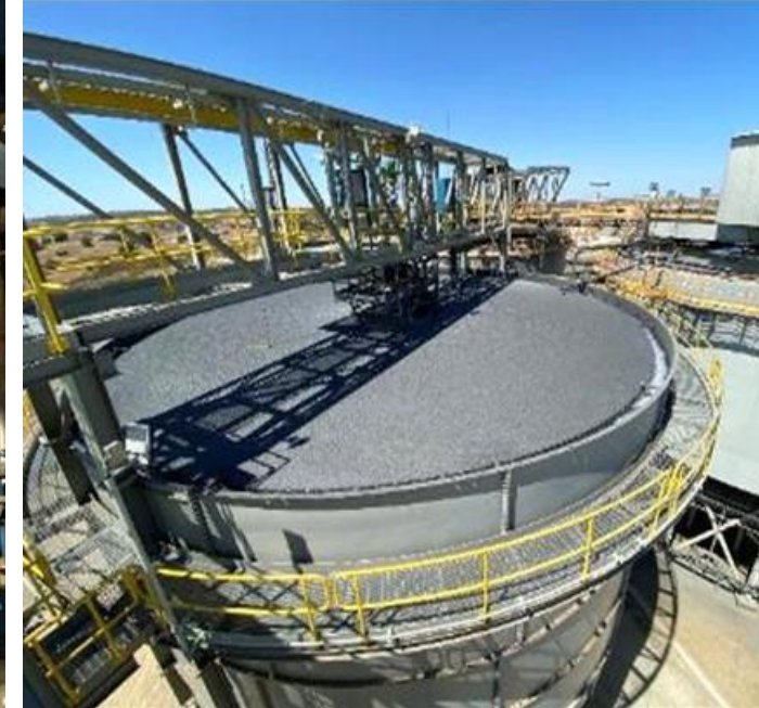
3 rd tailings paste thickener commissioned
