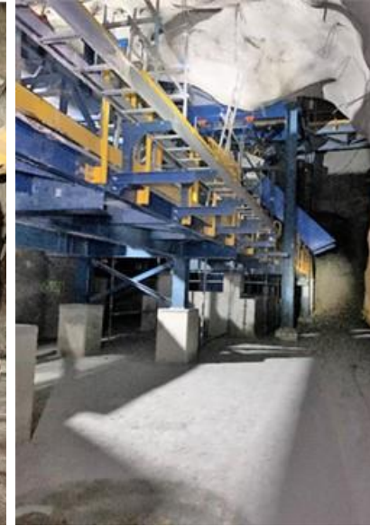
Installation progress on silos of 230 distribution level
