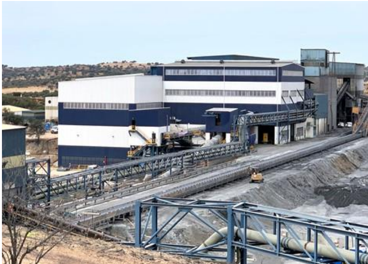
SAG and flotation buildings
