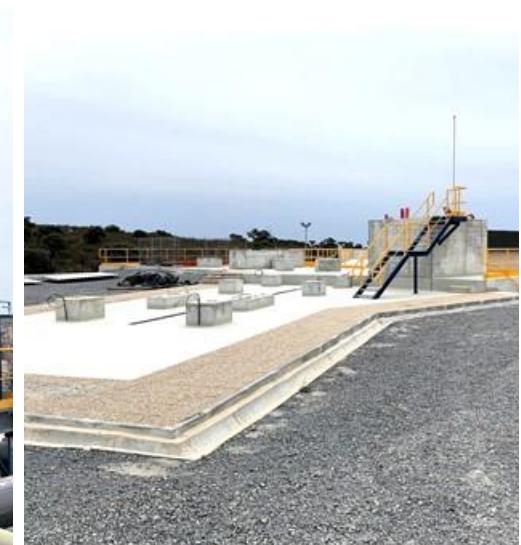
Ventilation raise 23 civil and electrical works completed
