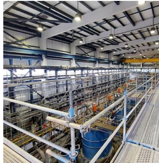
New flotation building
