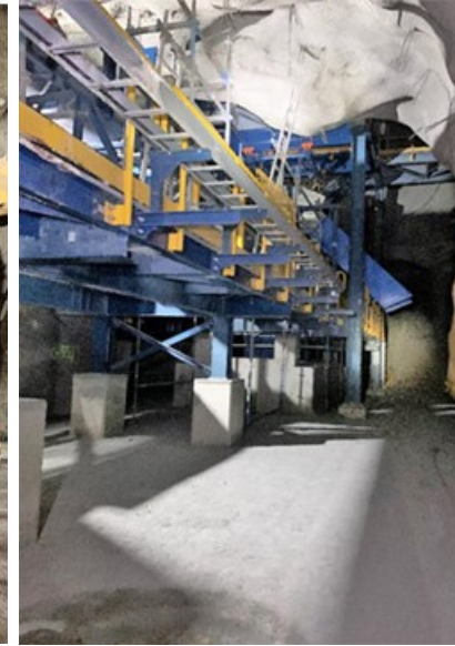
Installation progress on silos of 230 distribution level
