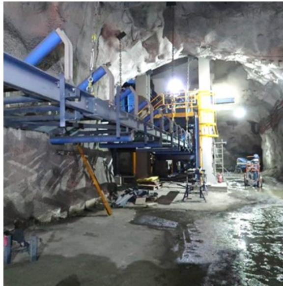
Silo and conveyor system installation on 650 skip loading level
