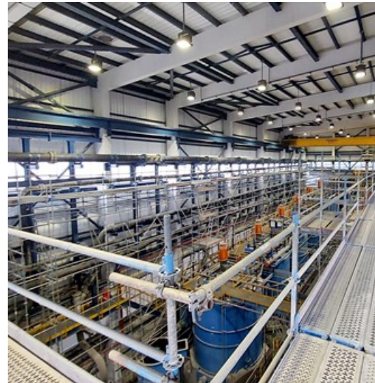
New flotation building
