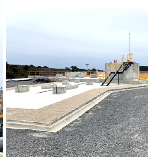
Ventilation raise 23 civil and electrical works completed
