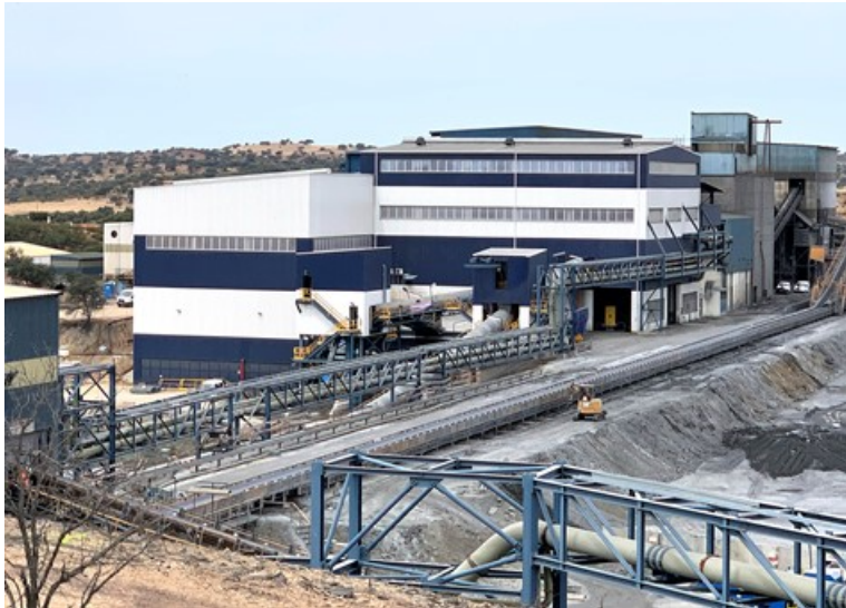
SAG and flotation buildings
