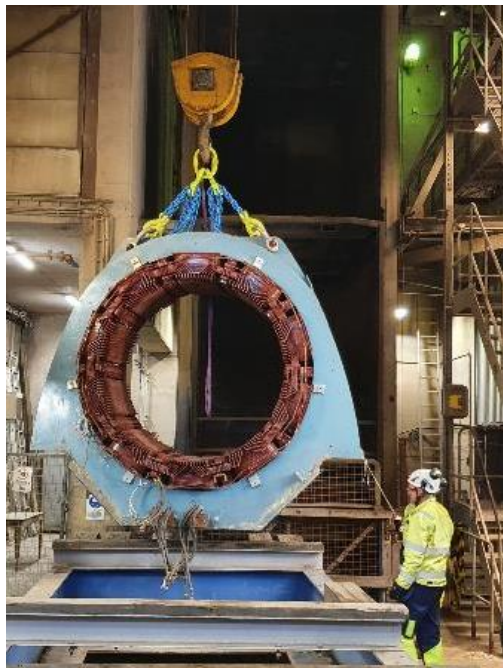
Maintenance work on P2 hoist motor completed November 2020
