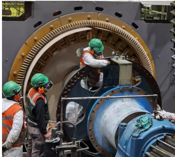
Installation of final ball motor in December 2020 to complete CMOP
