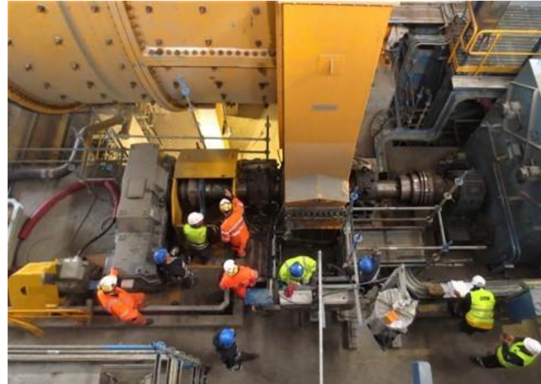
SAG mill commissioning work
