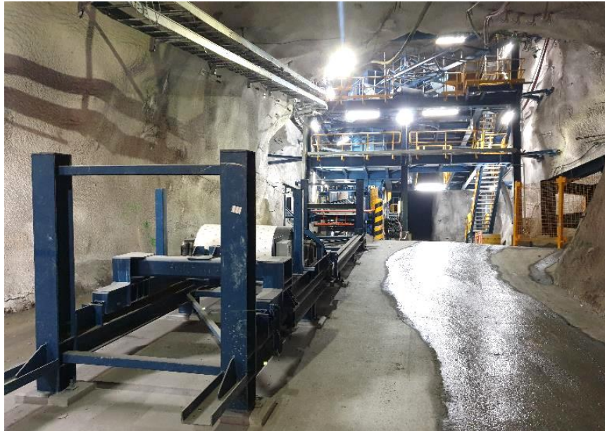
Installation of Transfer Station 3 ongoing
