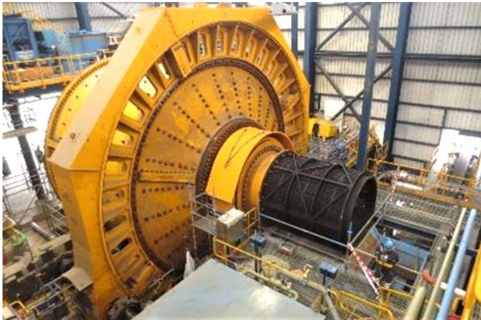
SAG mill motor and hopper installation
