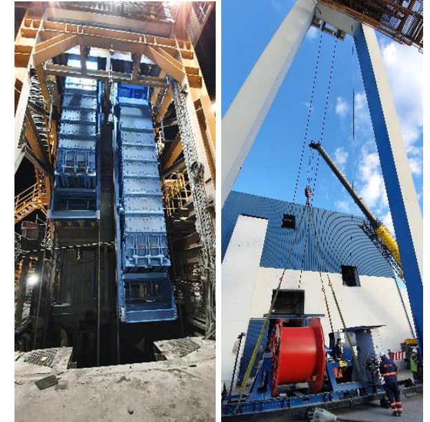
New skips and hoisting rope installed
