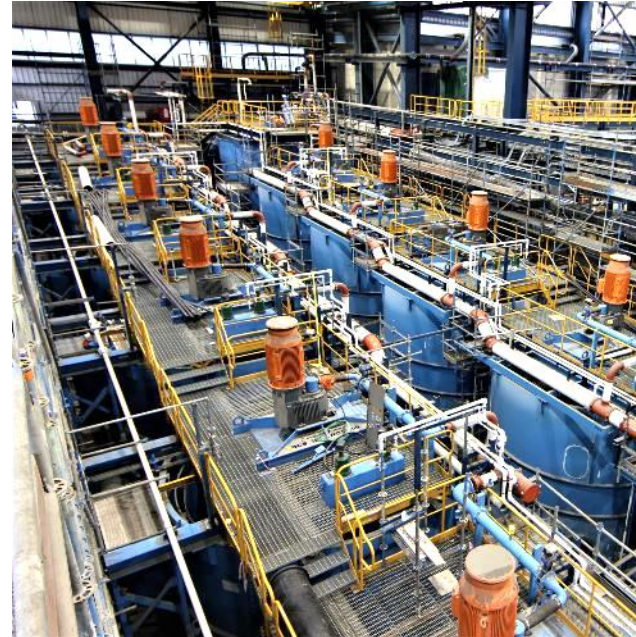
New flotation building piping installation
