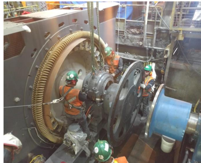
Candelaria Ball Mill 2 motor replacement during Q4/19
