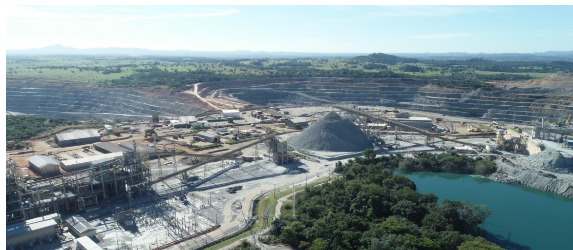
Existing crushed ore stockpile and crushing infrastructure in center and background
