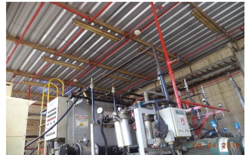
SAG / Ball mill lubrication system
