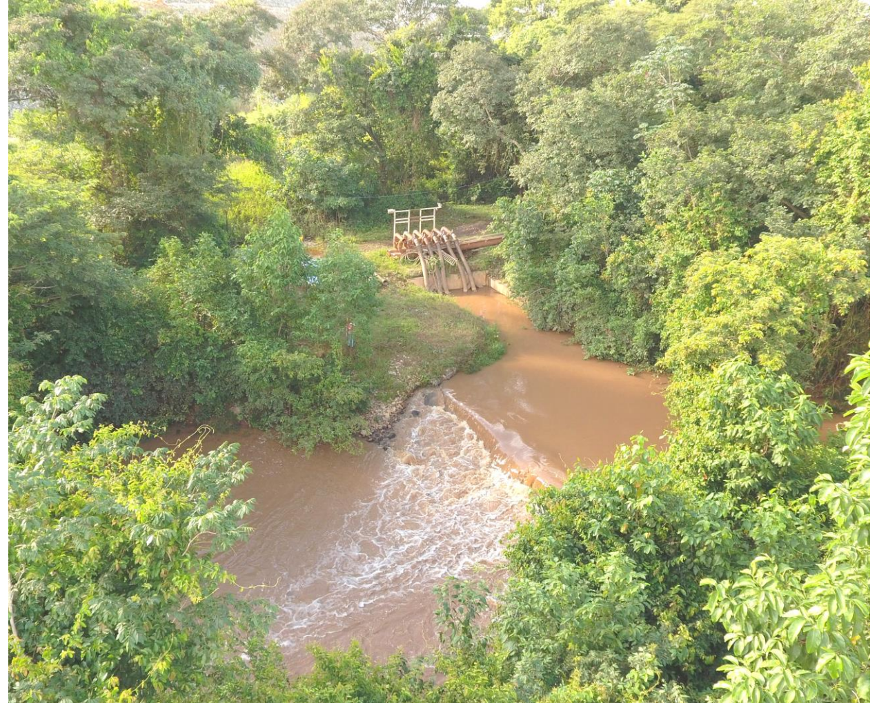
Water intake system Bois river
