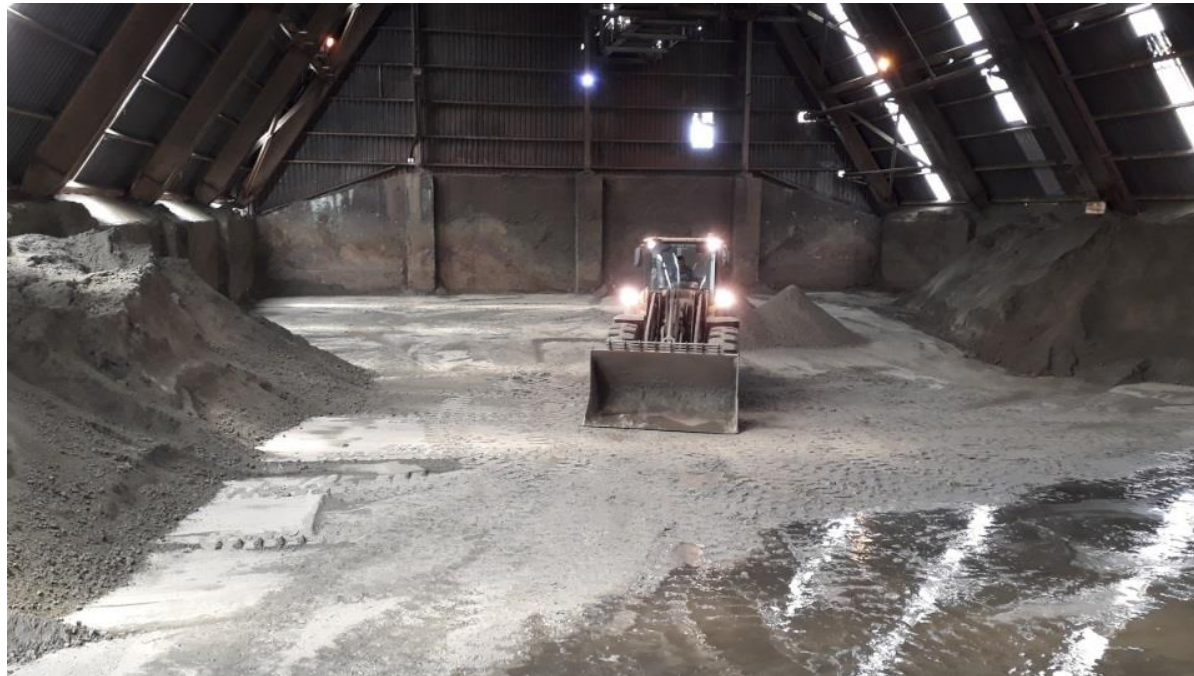
Concentrate storage shed; 6,000 t capacity
