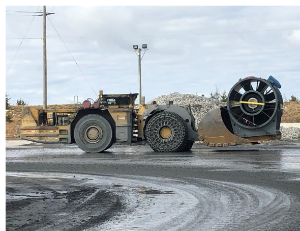
Eagle East main vent fan installation
