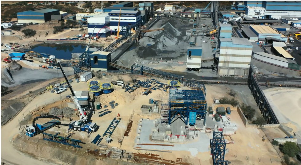
Transfer tower, pipe rack and conveyor construction
