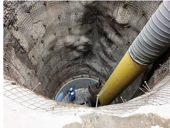
Silo G lining
