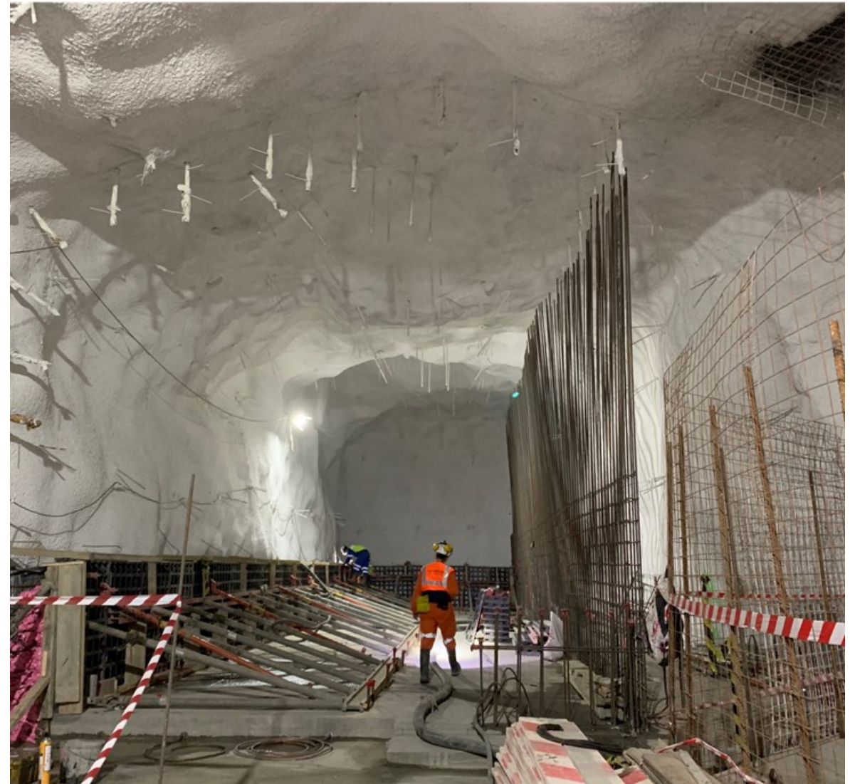
Development of Under Ground Electrical Room
