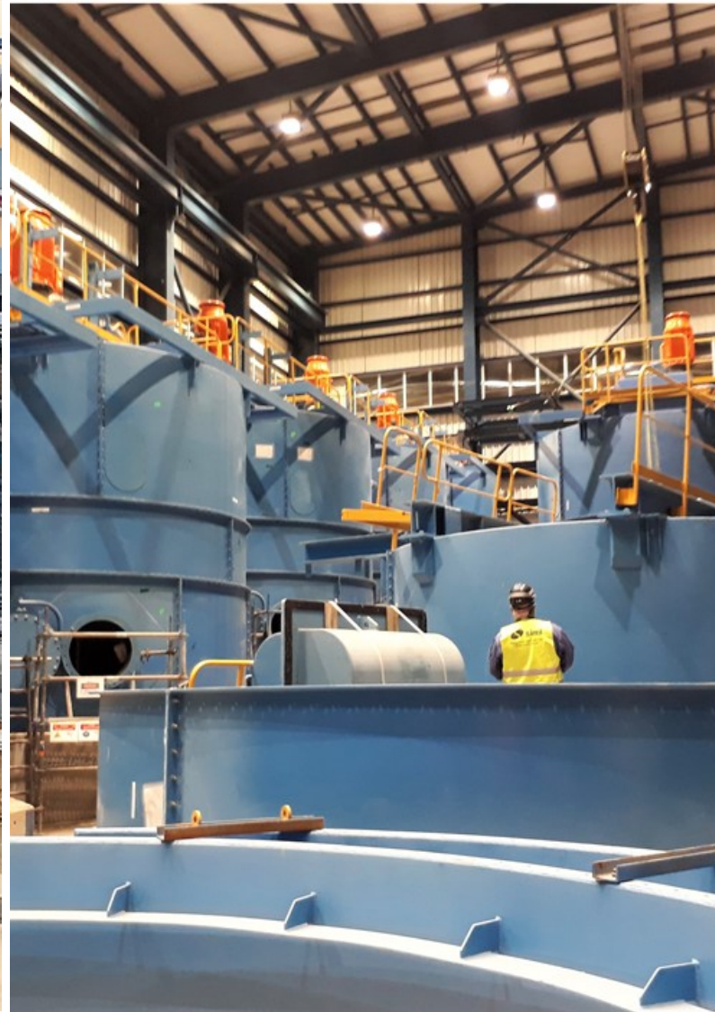
Flotation Cell Installation
