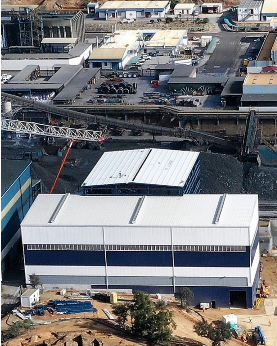
Flotation and Filtration Buildings
