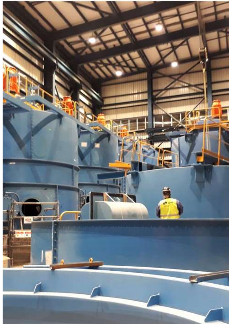
Flotation Cell Installation
