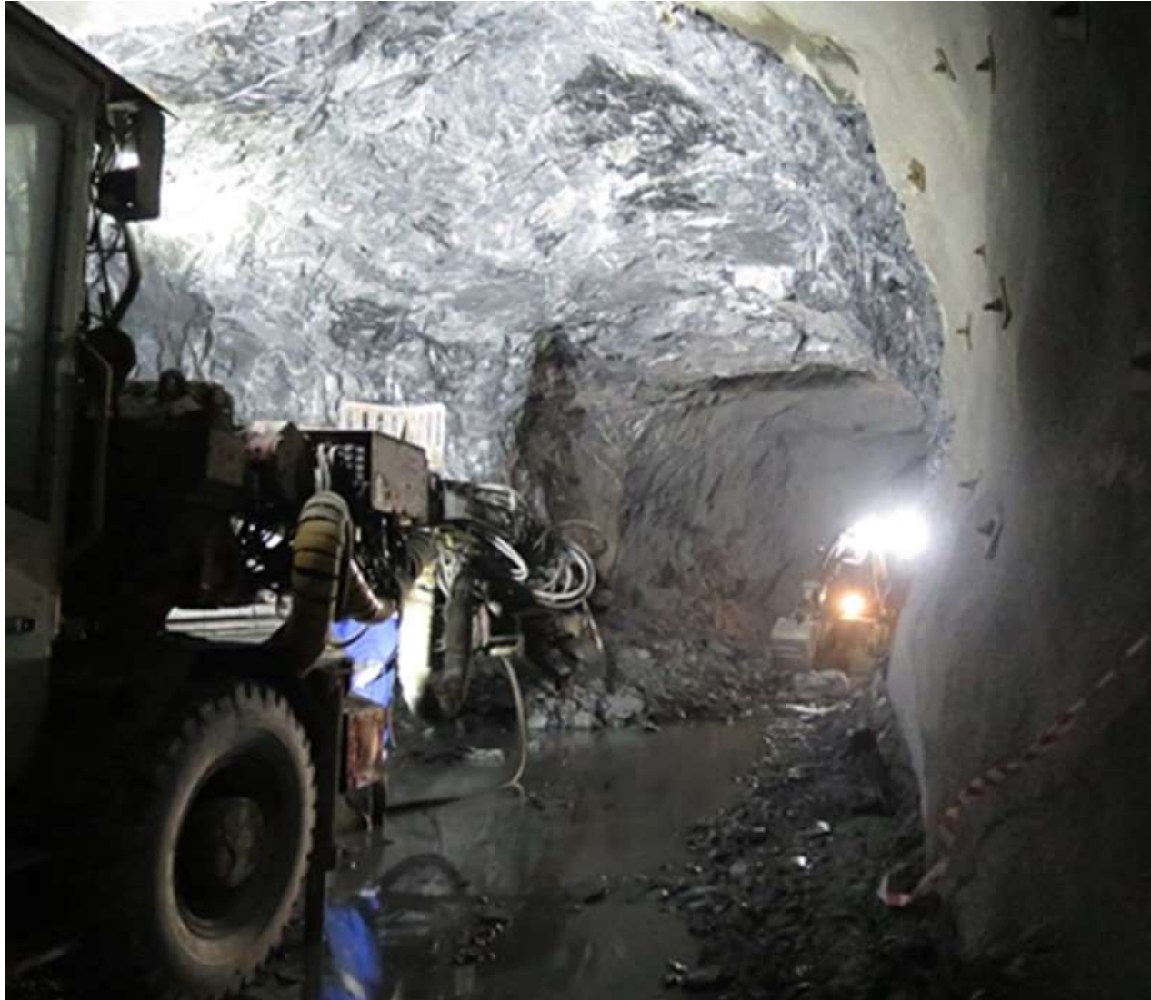
Breakthrough of Ramps 6 and 7
