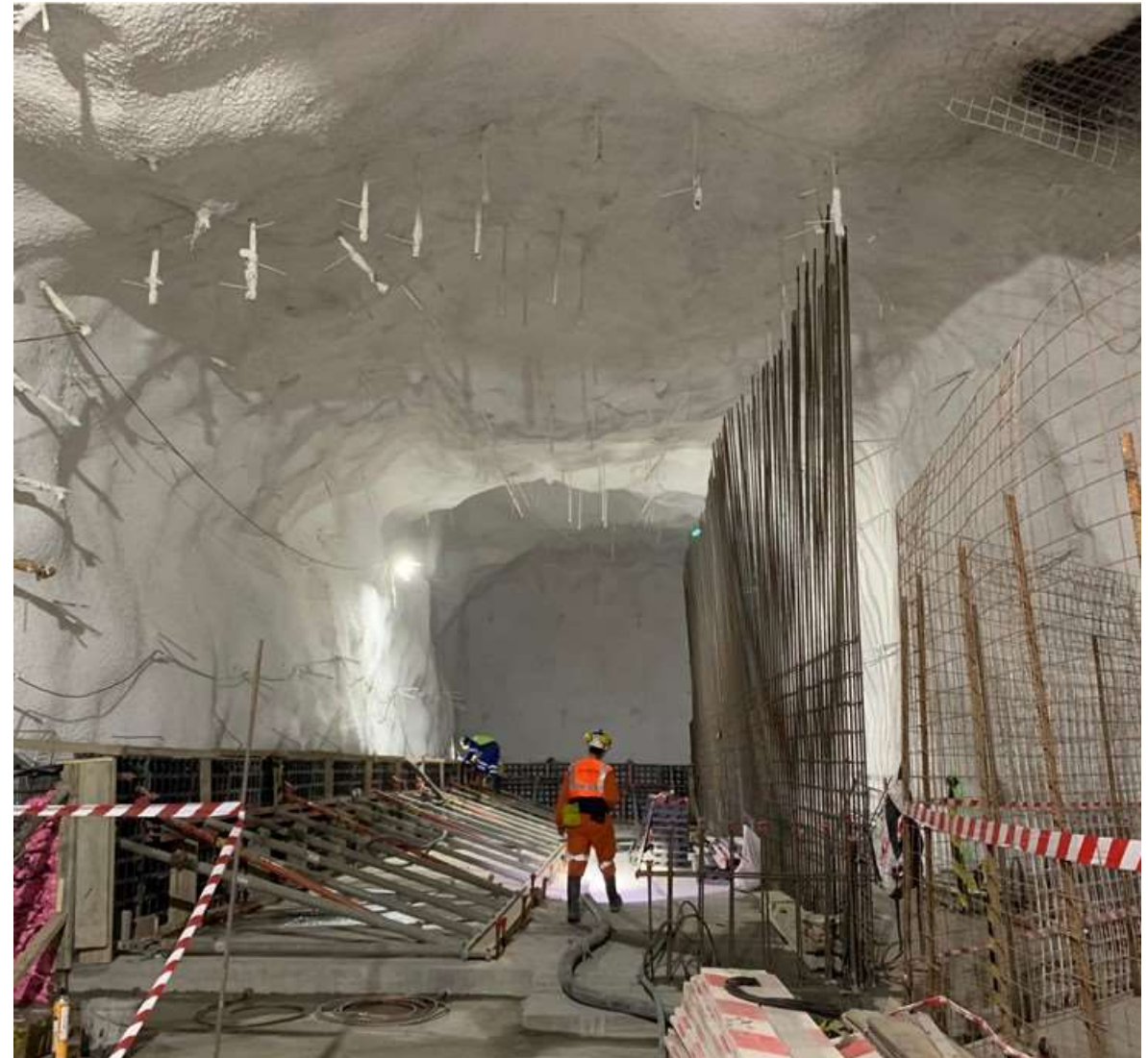
Development of Under Ground Electrical Room
